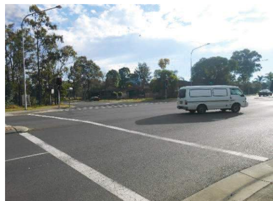
Figure 2.5: Quakers Hill Parkway/ Quakers Road Intersection (looking east)
